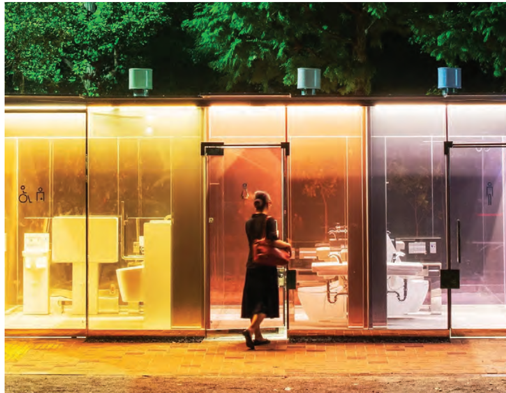
Precedent Example: Tokyo Olympics Restrooms
