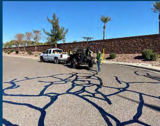
Crack Seal
