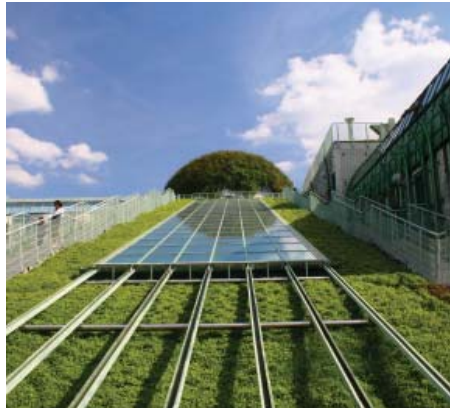
Photo 1.4.2 Green Roof/ Photovoltaic Panels
