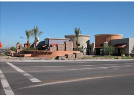
Santan Freeway Development
