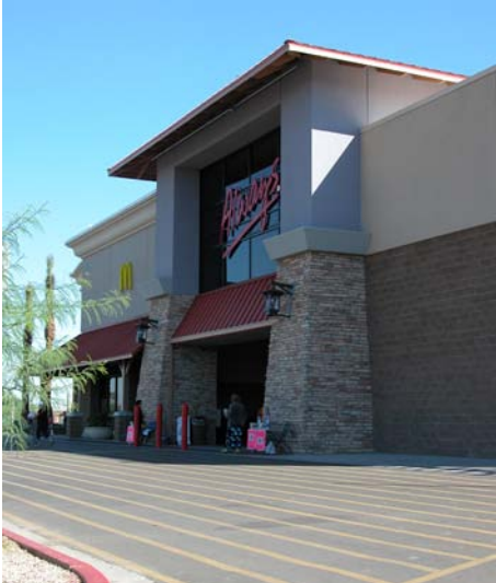
Santan Freeway Development
