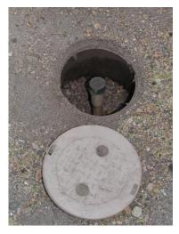
If your system has the threaded caps inside of pit boxes, unscrew the cap before turning the zone on. The water will be at a lower pressure and will fill the box with water. Just like the filters, they have hose threads, not pipe threads so use the short piece of garden hose to keep the box dry like with the filter flushing.
