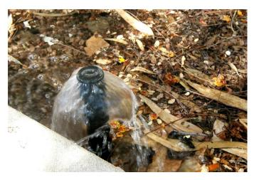
While the system is running inspect it for leaks or damage to the bubblers, risers, or piping. Timing the inspection to when the zone needed to run can allow you to run the full run time and make sure the water doesn't overflow from the berms.
