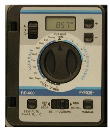
We run our irrigation at night so problems are often undetected. You want to turn it on during the daytime so you can observe the system when it is running. This is best done at the irrigation controller. This is a good way to verify that the watering schedule is correctly programmed for the season. Additionally, wiring problems will go undetected if the irrigation checks are done by manually opening the valves.
