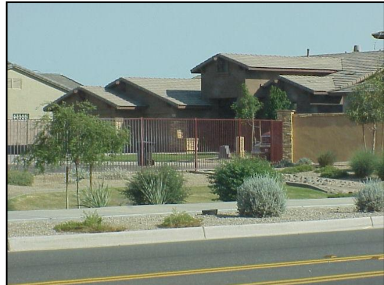
View fencing creates relief from solid walls.
